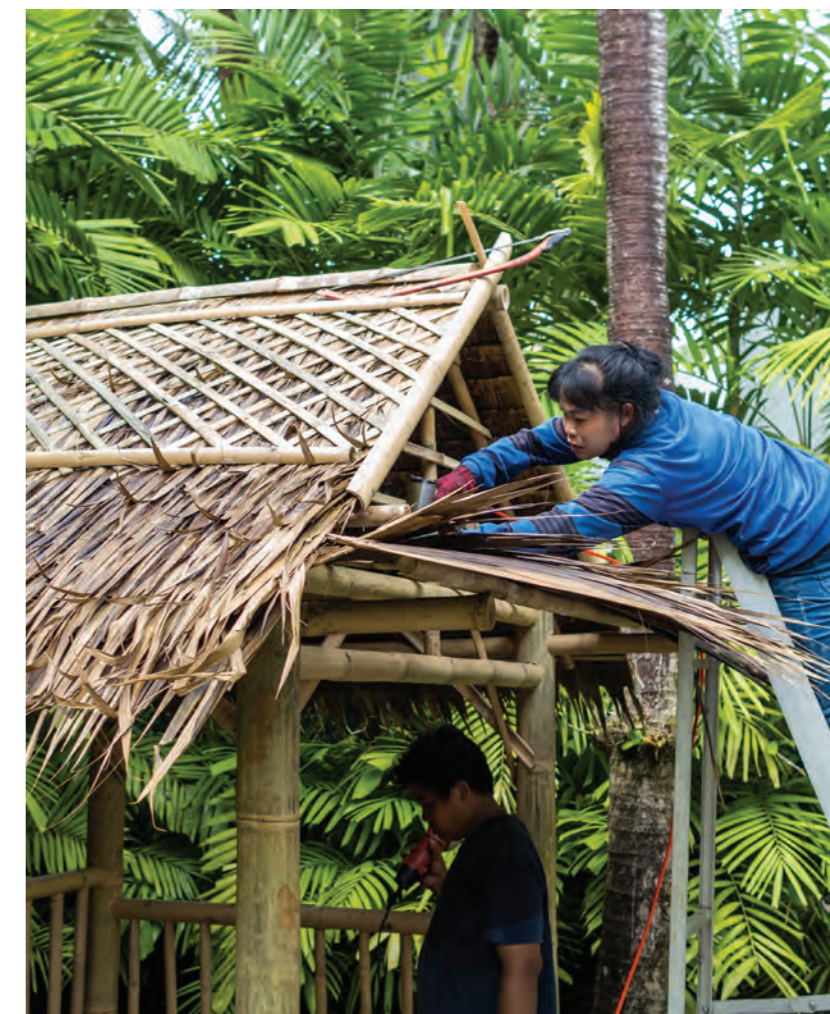
Building with Bamboo
